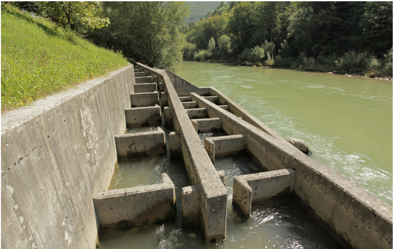
Fishways - such as this slot-style facility on the Steyr River, Austria - often fail to address the broader ecological impacts of fluvial barriers and typically benefit only a limited number of species. © SPARE (INTERREG Project) / Simone Sozzi / Water Alternatives, CC BY-NC 2.0
